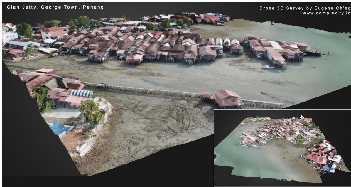
Figure 3. Site 3D survey and capture of George Town's Clan Jetty
